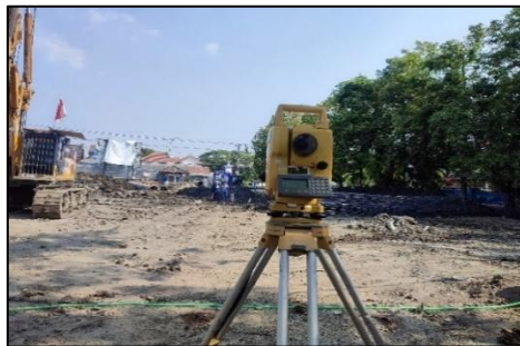
Gambar 3. Penentuan Titik Bored Pile
